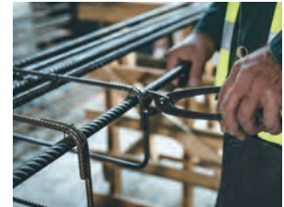
Rebar Installation
