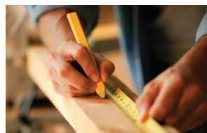
Minor Carpentry Work
