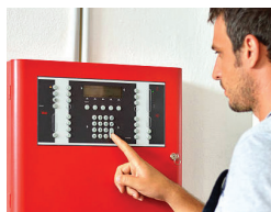
Fire Alarm Installation & Repair
